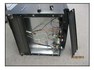
6. Locate the thermocouple and remove from back of gas valve with 5/16" wrench.
