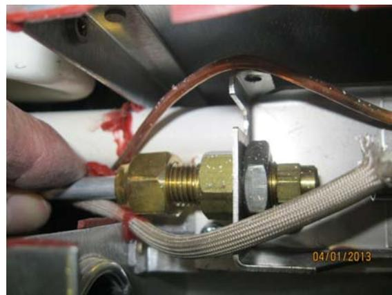
7. Tighten each connection with a back up wrench
